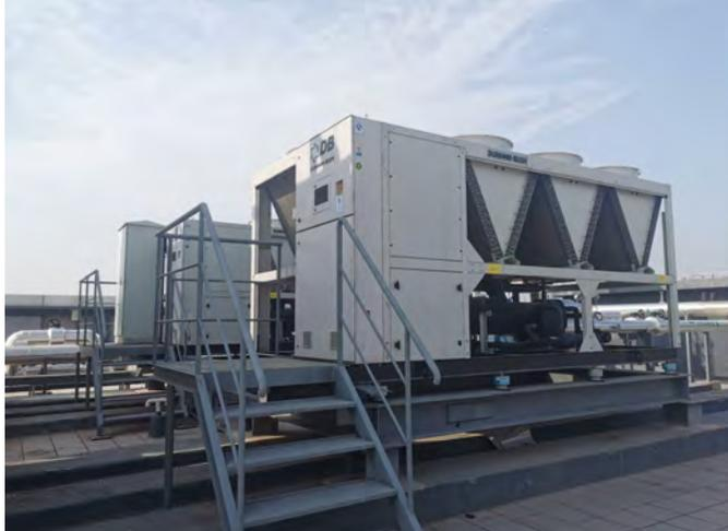
A large, white, industrial-grade screw compressor unit with a metal staircase leading up to it, located on a rooftop platform.          |
